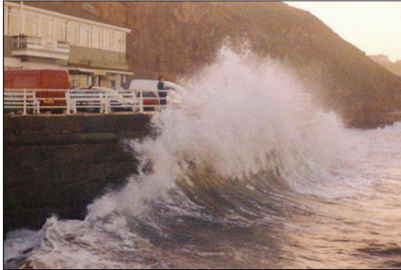
Figure 1.1: Wave overtopping of a harbour wall. Whitby, United Kingdom. (Photograph by the author)
